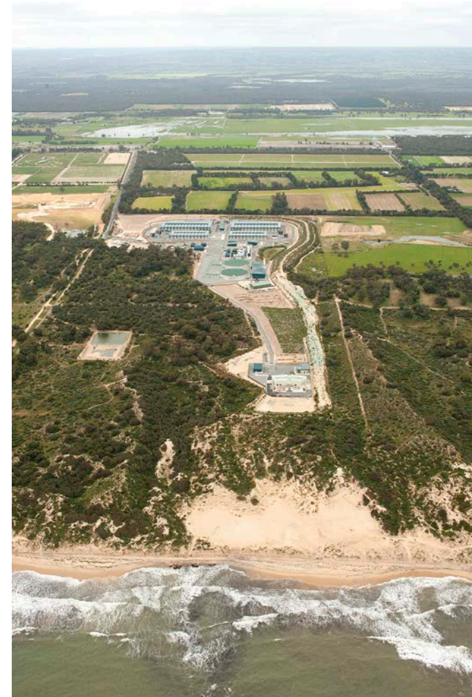
Figure 5: Southern Seawater Desalination Plant (Source: Water Corporation)
