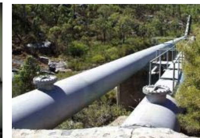
Distribution systems protection (including chlorine residuals)
