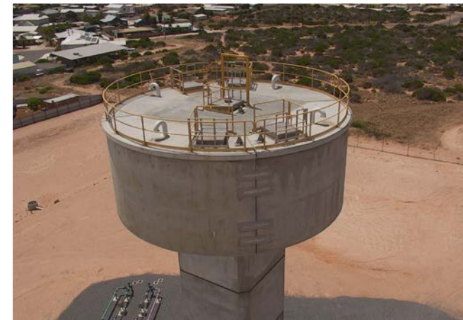
Figure 28: Denham elevated tank
