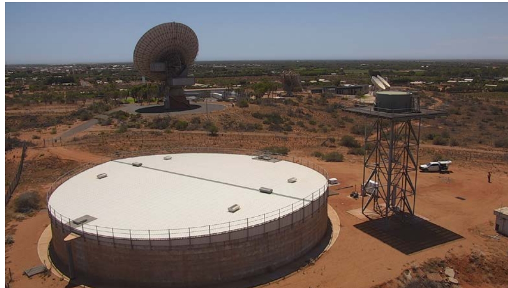
Figure 3: Carnarvon elevated and ground level tanks – image taken by drone (see Case Study - The use drones for catchment management, page 33)
