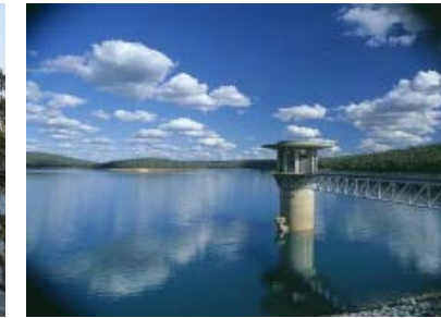
Large reservoirs with long detention times
