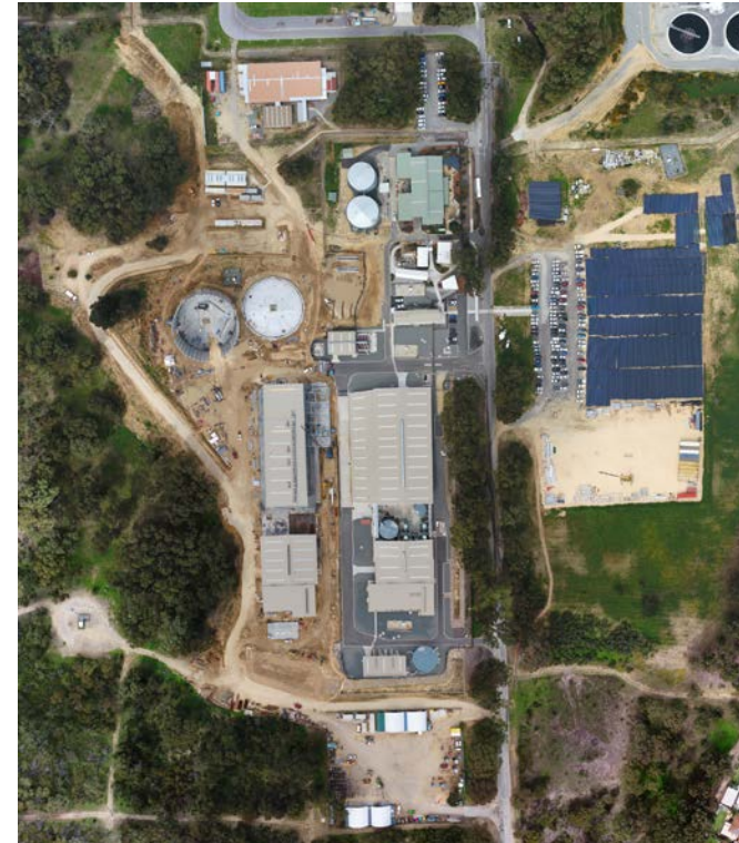
Figure 15: Birds eye view of GWR Stage 2 under construction
