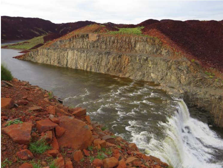
Figure 30: Harding Dam overflowing
