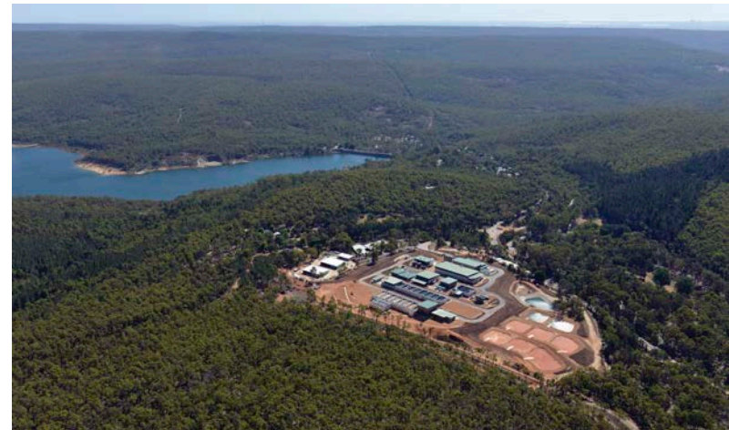
Figure 1: Mundaring Water Treatment Plant (Source Water Corporation)
