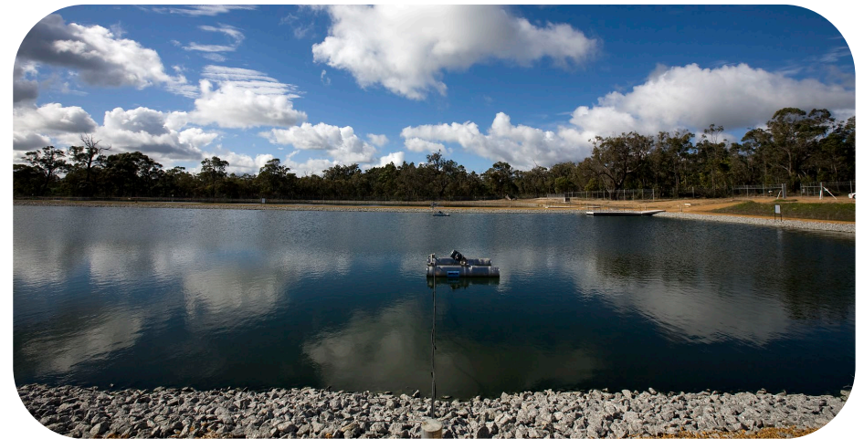
Figure 2: Mount Barker WWTP – wastewater treatment pond
