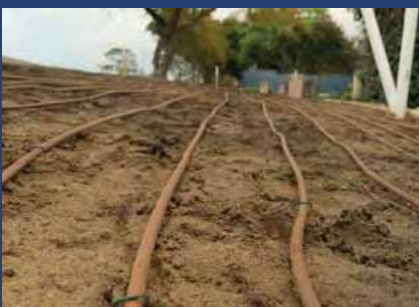
Drip irrigation installed
